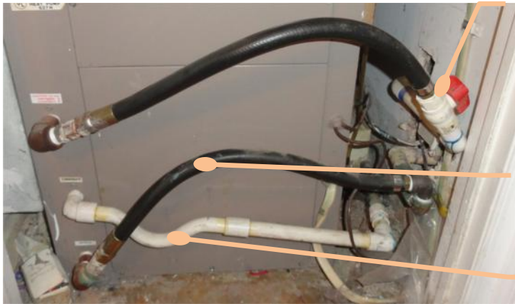
Figure 6. Unit Heating and Cooling System with Updated Valves and Hoses
