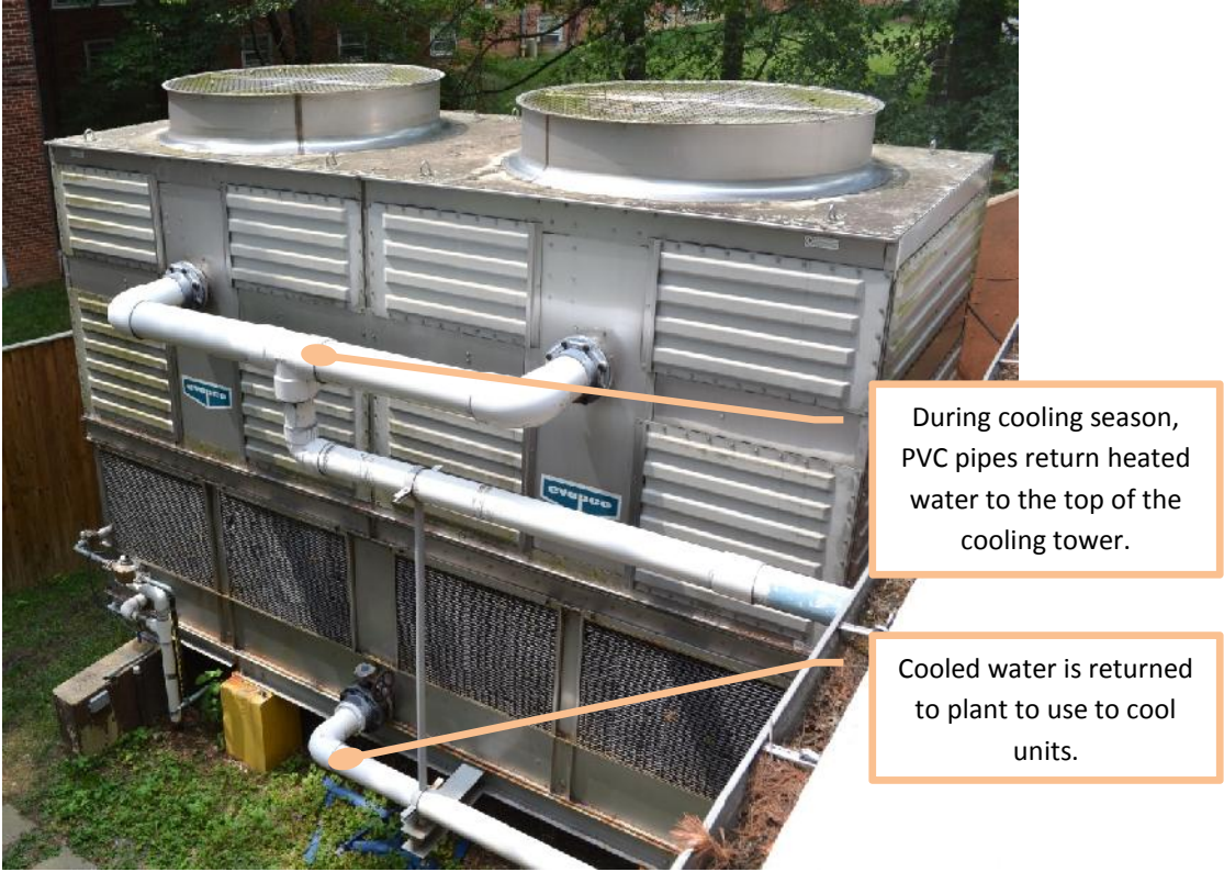
Figure 15. Electric motors power cooling fans.
