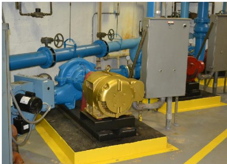
Figure 11. Electric motors power the pumps that circulate the water in the loops.
