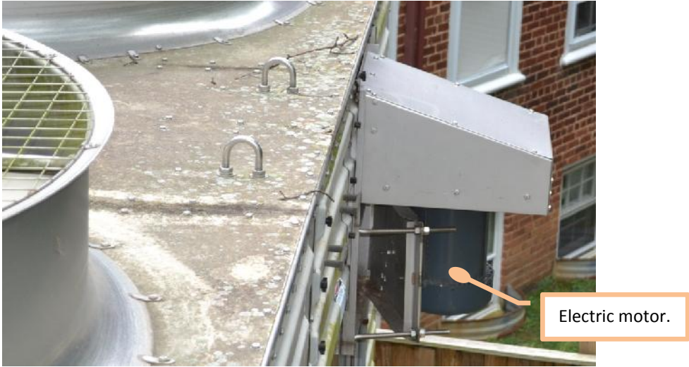
Figure 15. Electric motors power cooling fans.
